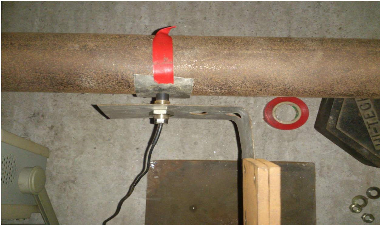
Fig: Use of Proximity Sensor
