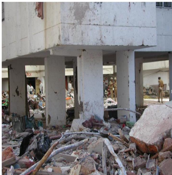
Figure1.2: Collapse of structure at Ahemdabad due to earthquake
