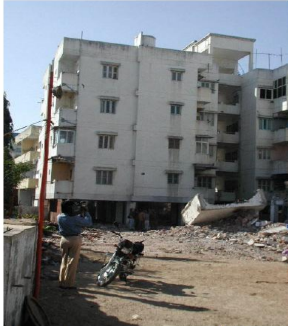
Figure 1.1: Collapse of structure due to earthquake
