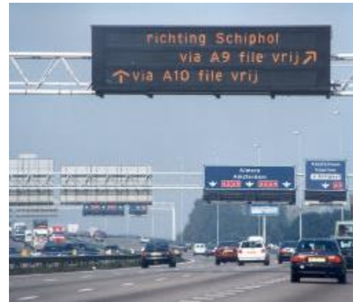
Figure 1.8: Informative Rerouting Messages
