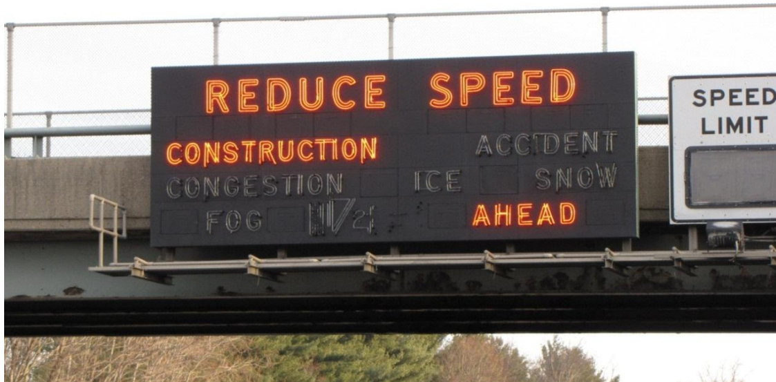
Figure 4-33: Variable message sign
