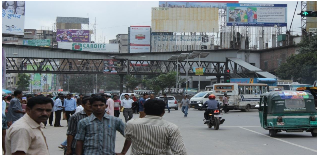
Figure 4-11: Presence of foot over bridge
